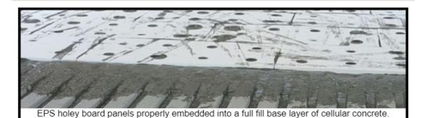
A void-free, full and adequate slurry layer and full underside contact with the embedded EPS panels shall be considered required for meeting an assembly's internal fire-resistant and wind uplift ratings.
